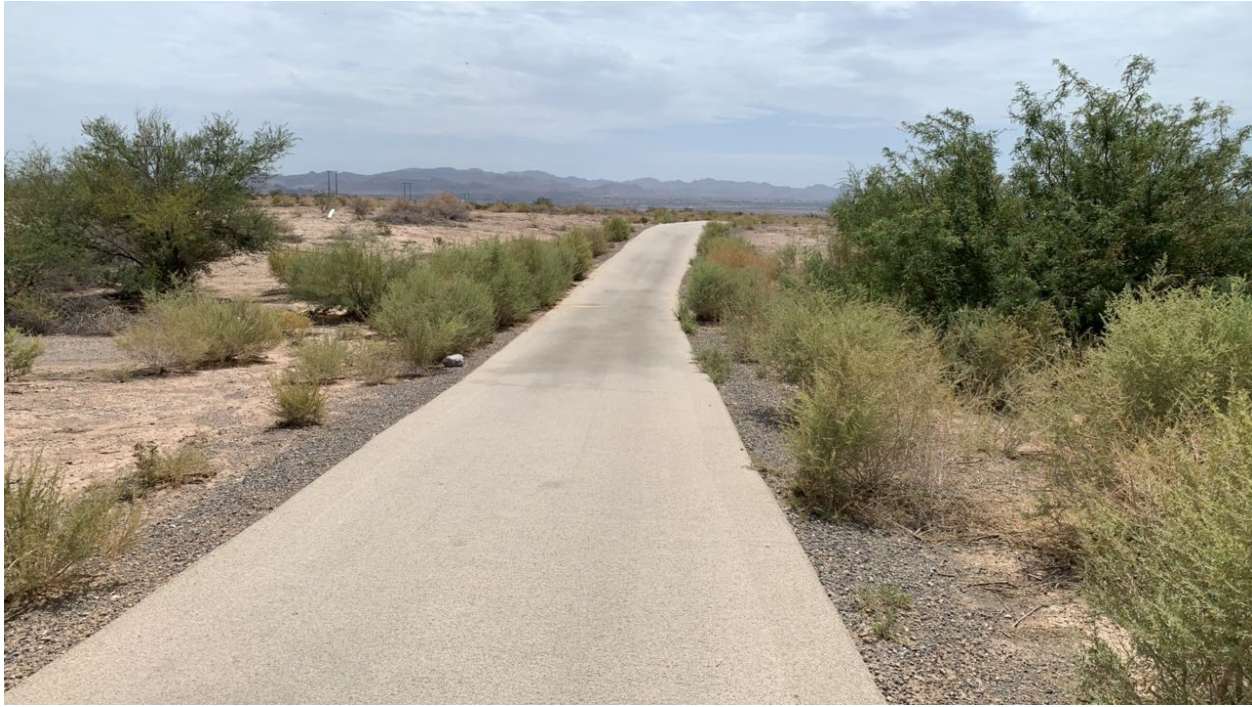
Figure 28. Photo of Downstream Upper Diversion North-2.
