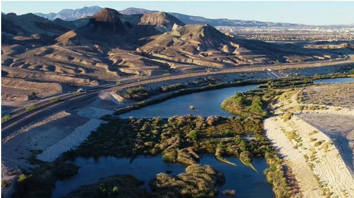
Figure 29. Aerial image of Three Kids Weir which was constructed in 2015. This weir site is the largest at 4.74 acres. Photo taken in 2020.
